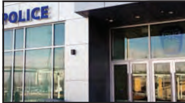
SQUARE ONE • COMMUNITY STATION 100 City Centre Drive • Mississauga
